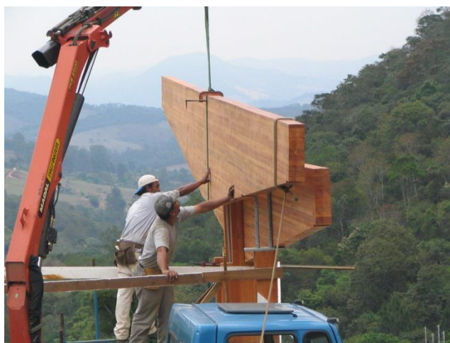
Figure 28: Haras Polana, glulam beams at work site
