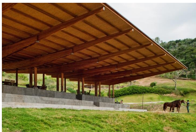
Figure 29: Haras Polana, 12m cantilever
