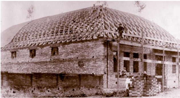
Figure 10: Wood segmental-lattice vaults, made by Hauff in 1927
